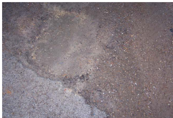
Area of asphalt decomposition
