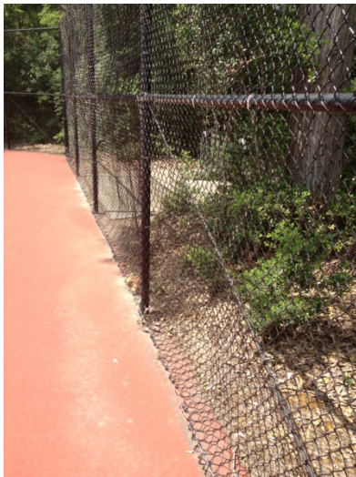
Typical damage to the Meadowlake Tennis Court fences
