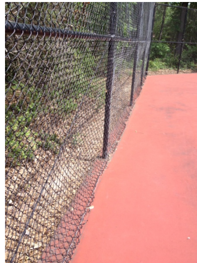
Typical damage to the Meadowlake Tennis Court fences
