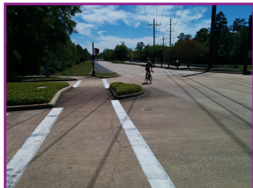
Figure 4.7: Bicyclist forced to use vehicular lanes due to bulb out issue in shoulder & curvature of shared use path
