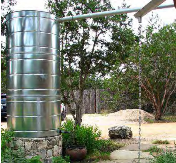
Rainwater harvesting system with landscaping.
